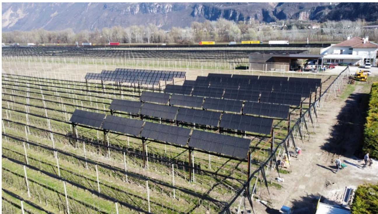
Figure 2.1 Agri-PV demonstrator in Bolzano (IT).
