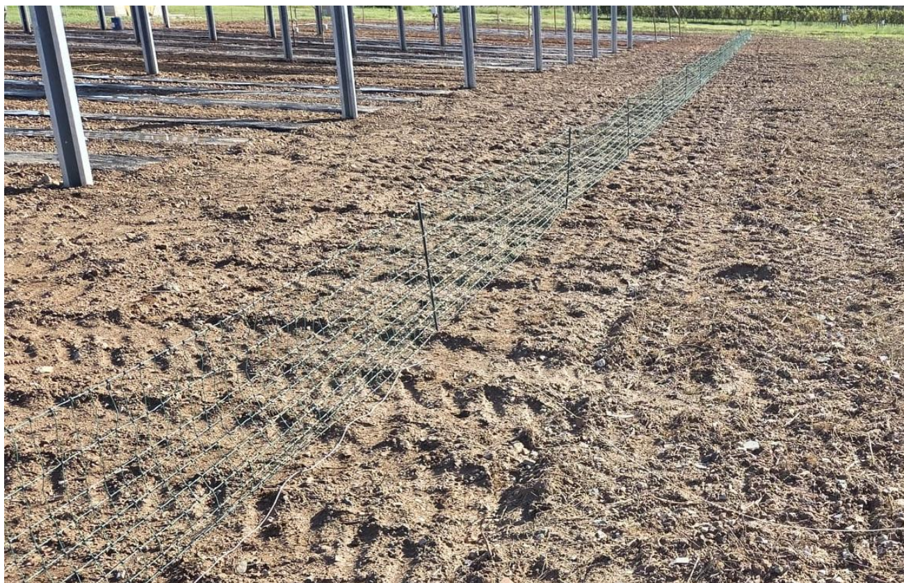
Figure 3.11 Installation of perimeter fencing for crop protection around the agrivoltaic structure.
