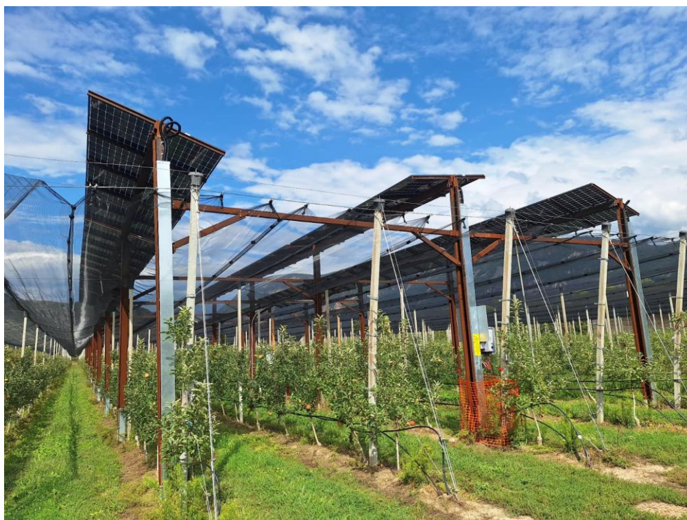
Figure 2.9 Hail nets installed in the new plant orchard in Bolzano demo.
