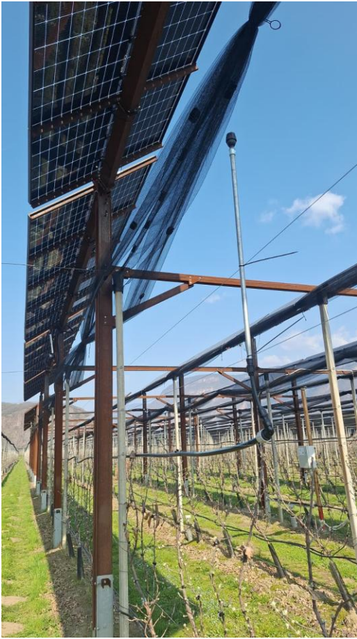
Figure 2.8 Anti-frost system installed in the Bolzano demonstrator.
