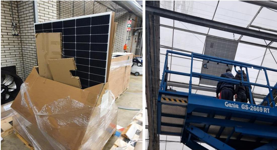
**Figure 133:** PV panel to be installed (left) and the first PV panel being installed (right)
